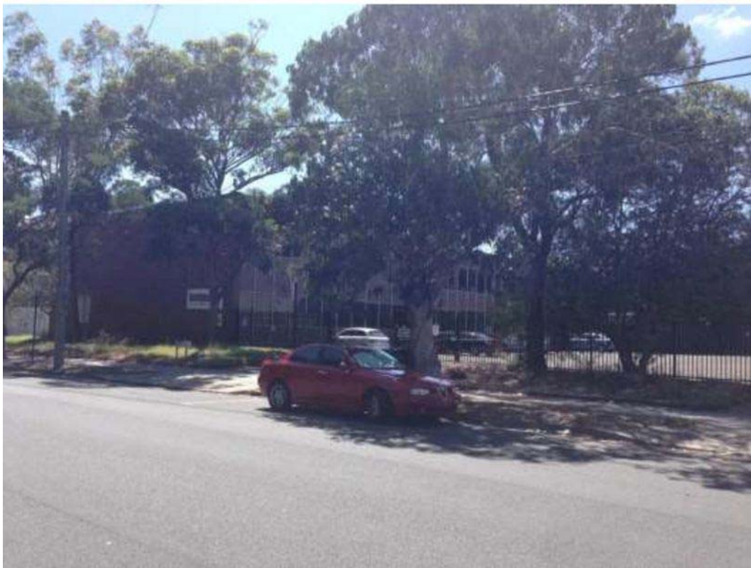
Figure 6: Rosebery Avenue frontage (southern end)
