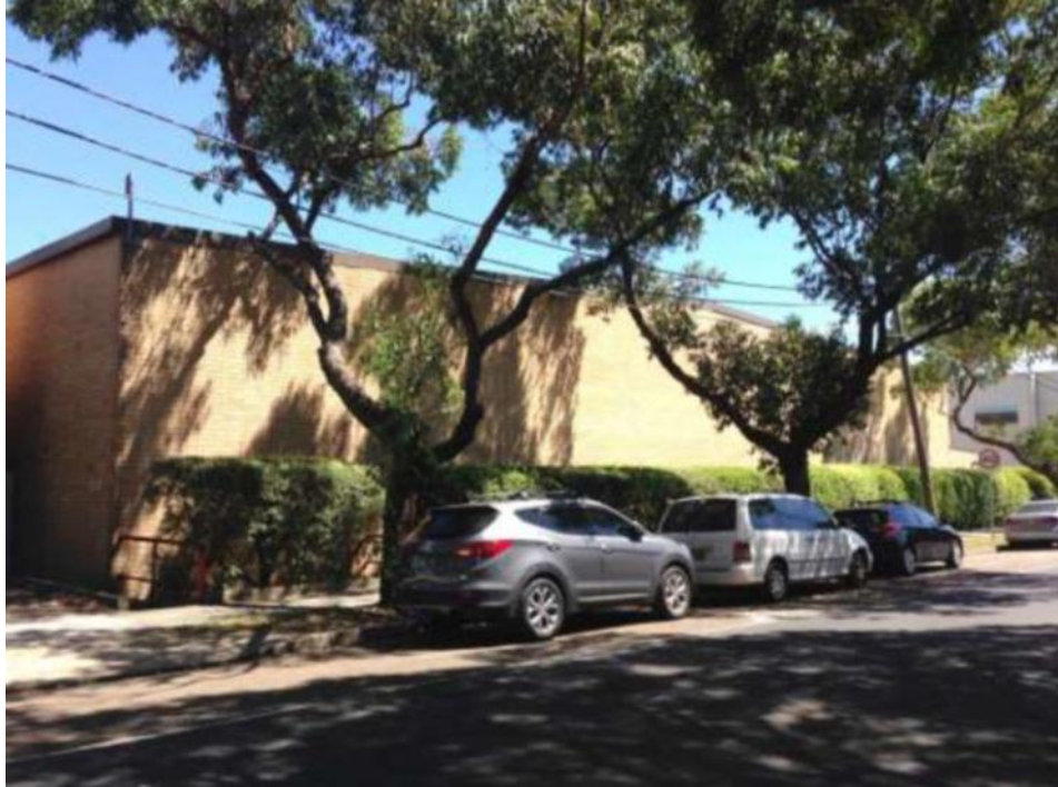
Figure 9: Two storey warehouse adjoining the northern boundary Dalmeny Avenue
